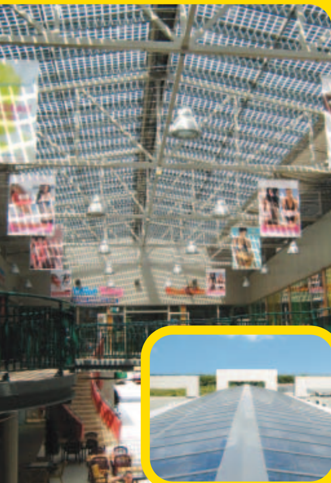
© Photos Solar Electric Guadeloupe
