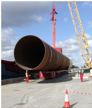
Monopile delivered to harbor
