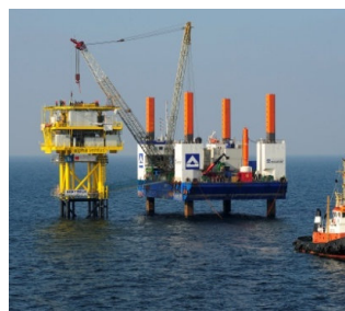
Transformer topside installation
