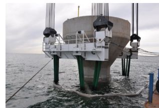
1,300 ton foundation being positioned
