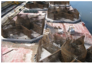
Construction of the steel formwork
