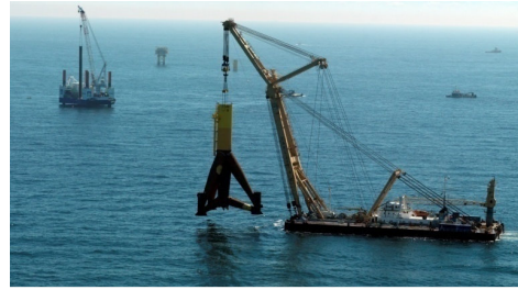
Heavy-lift crane ship during foundation installation
