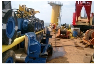
Cable pulling to foundation
