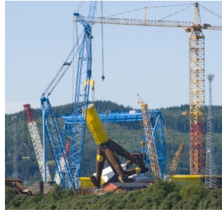
Tripod up-ended for shipping
