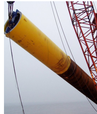
Monopile being up-ended for installation
