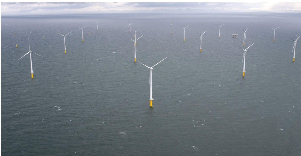
Picture taken at E.ON Offshore Project - Robin Rigg (UK, 2009)
