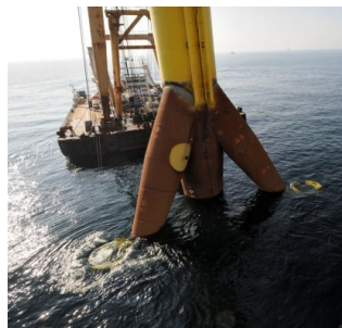
Tripod foundation being lowered to seabed
