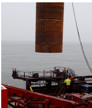
Pile gripper for exact pile positioning
