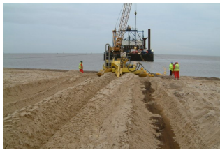
Cable plowing on shore
