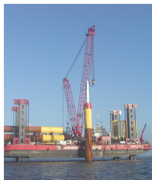
Pile hammer (300t of force) driving monopile
