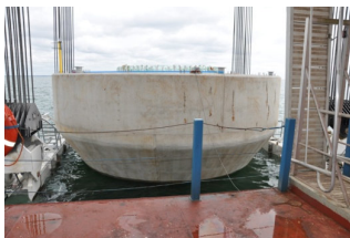
Foundation being lowered to seabed
