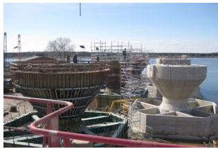
Foundations are cast in concrete
