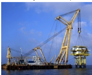
Heavy-lift crane ship
