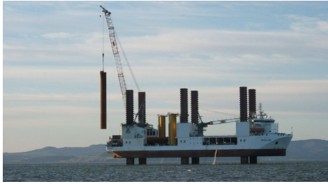
Jack-up crane vessel during foundation installation
