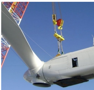
Turbine nacelle being positioned on tower
