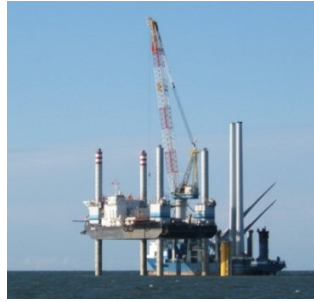
Offshore installation of turbine tower
