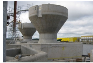
Completed gravity foundation
