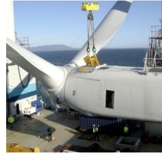
Turbine nacelle being lifted
