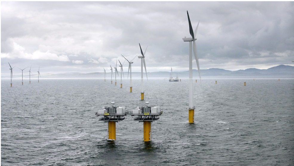
Picture taken at E.ON Offshore Project - Robin Rigg (UK, 2009)
