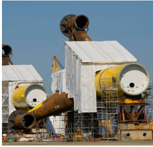
Tripods being welded in Norway
