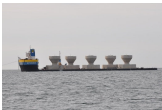
Foundations being shipped to site
